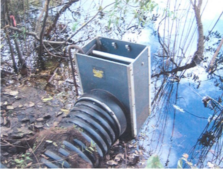
10x16 rectangular riser (10" above outlet top) discharging through 12" plastic corrugated pipe
